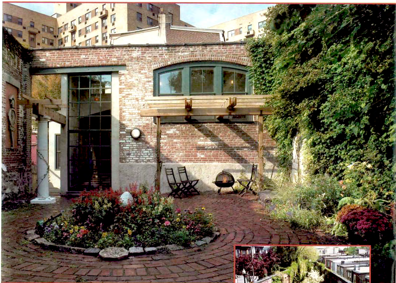
Above: New and old blend where an enclosed garden meets an addition to a Fairmount rowhouse. Inset: The back yard before construction.
